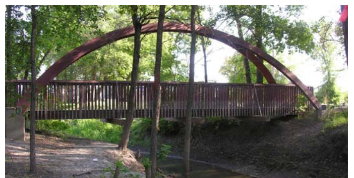
Two building rafters suspending a bridge about 60 ft long
